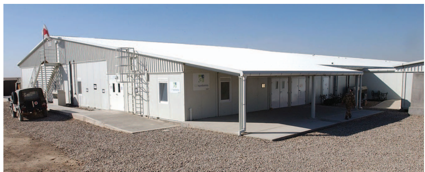
Figure 1 The 'New Build' Camp Bastion Hospital, when opened on 9 February 2008, showing the casualty reception area (Defence Images).
